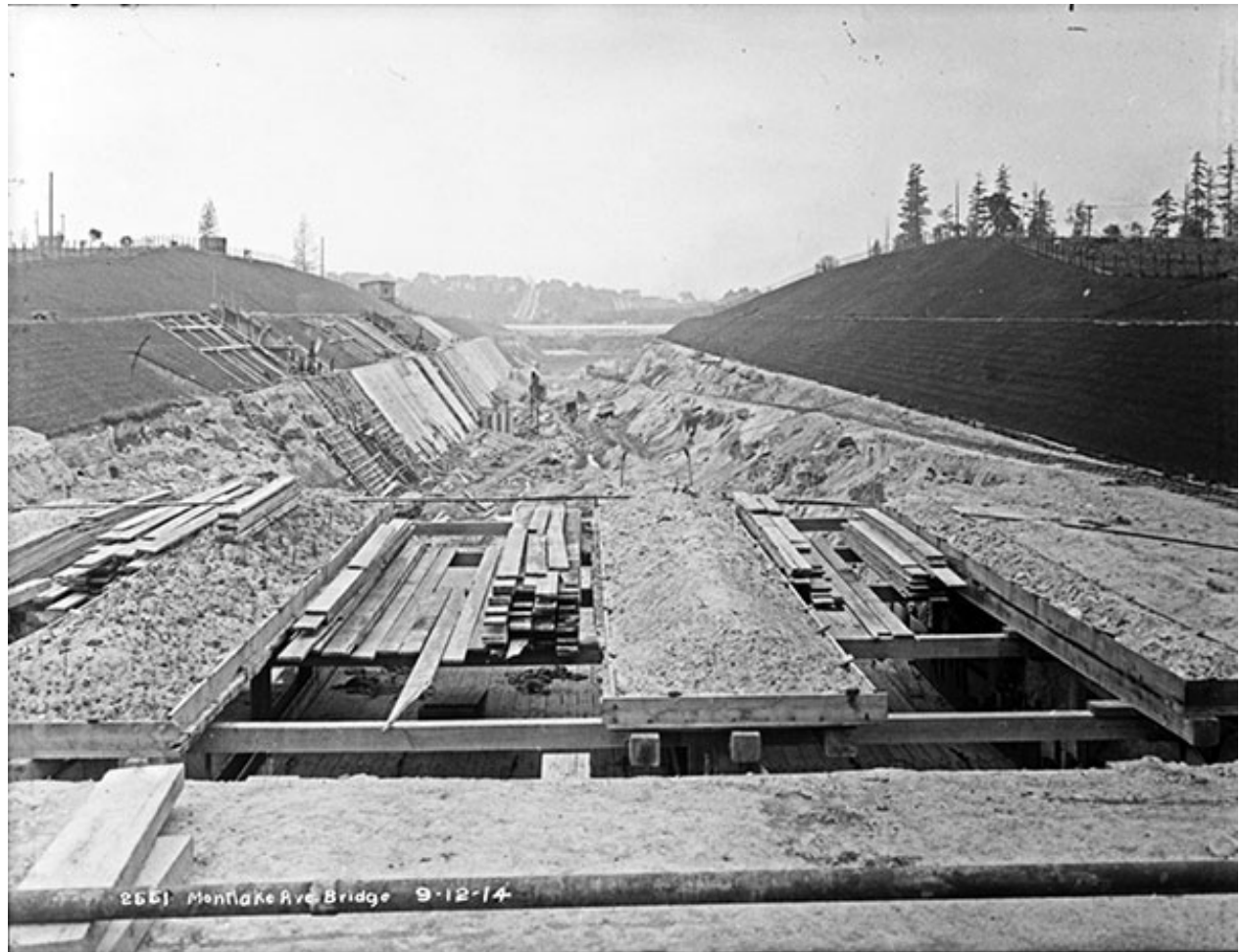
Looking east at Montlake Cut construction, Seattle, September 12, 1914.
