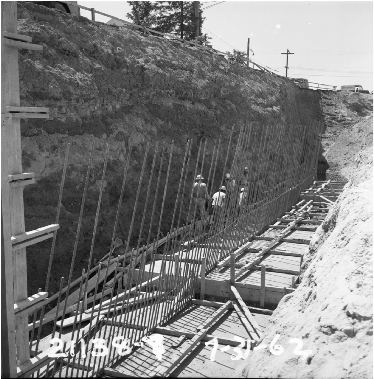
Seattle Municipal Archives. Montlake Interchange . 1962. Photo Number 72827
