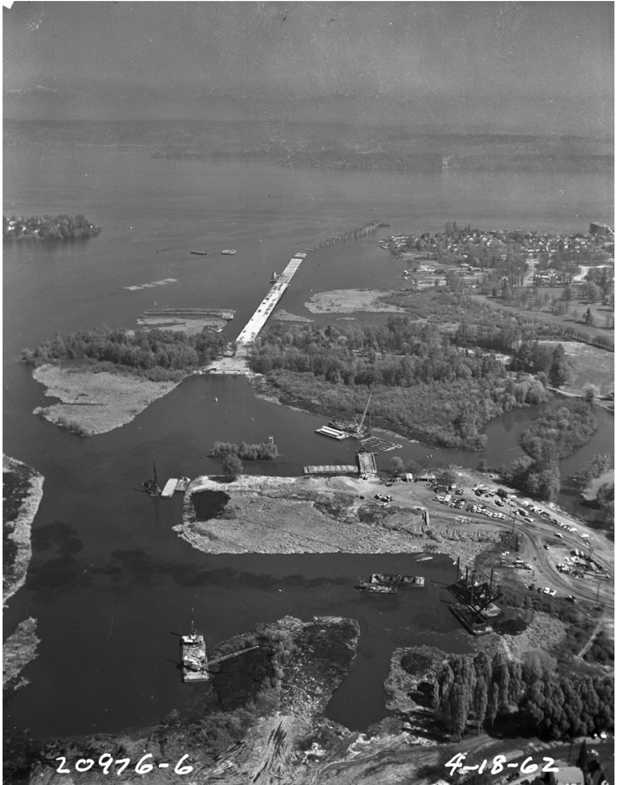
Seattle Municipal Archives. Montlake Interchange . 1962. Photo Number 71032
